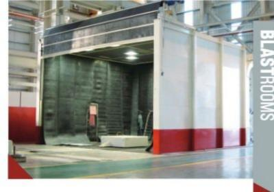
The recovery of the abrasive is through our W Series pneumatic conveying recovery floor and the different abrasive types are automatically separated into 2 separate storage hoppers ready for reuse. The recovery system is fully inter-locked to prevent cross contamination of the different abrasive types.
